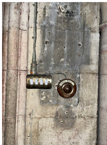
Figure 14 – Example of installation of electrical lighting in present day (Author's Own, 2024)
